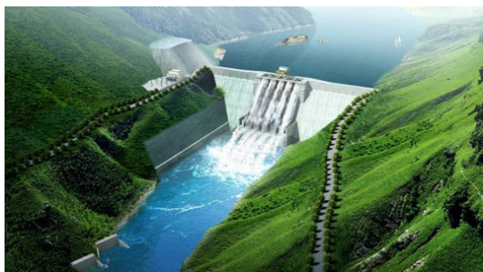
Tuoba Hydro-Power Station. 2015. Tuoba Hydro-Power Station, n.p
